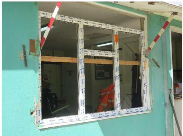
The new window frame
