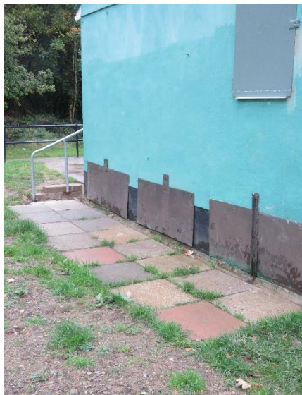
Pathway at the east of the building
