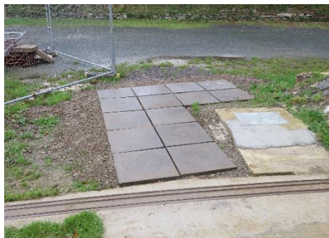
Pathway at the west of the building
