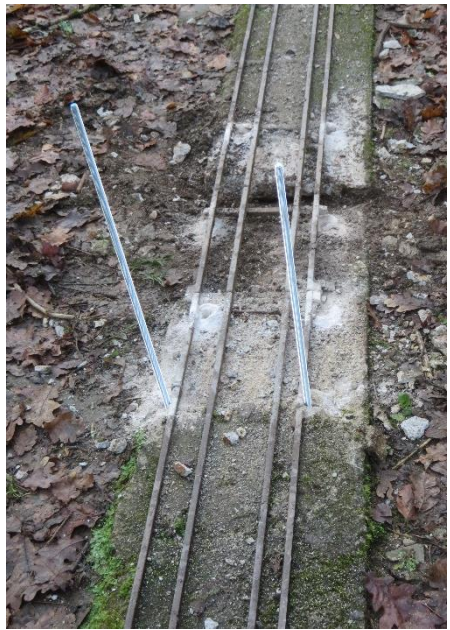
Another spot repair in progress
