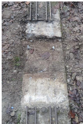
A new section is required to bridge this gap
