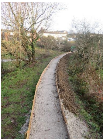
Track base approaching the bridge being prepared
