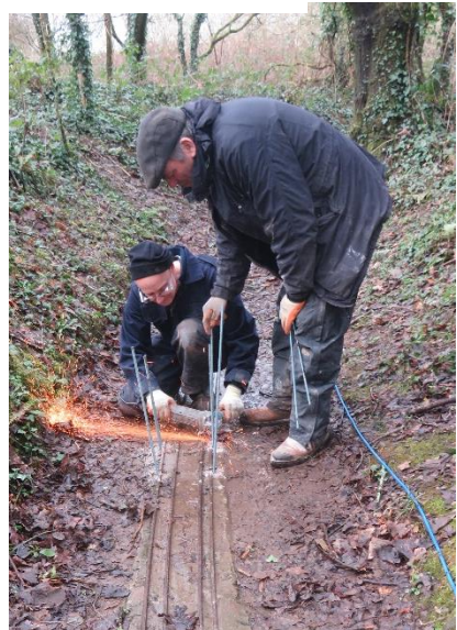
More spot repair action
