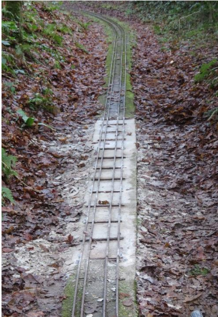
Track - spot repairs in progress
