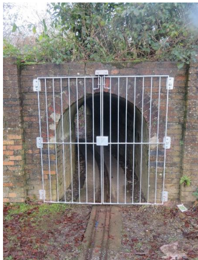
Completed tunnel gates - there is another set at the other end!
