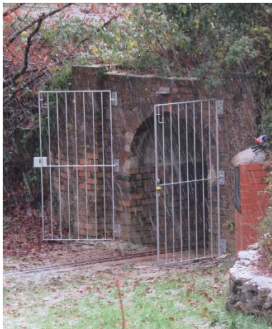
Tunnel gates being fitted in a hailstorm
