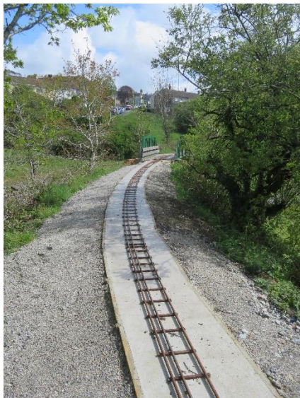
Delivered to site
