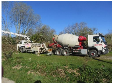
For the arrival of the concrete
