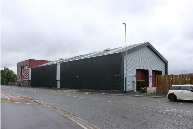
The New "Tin Shed"
