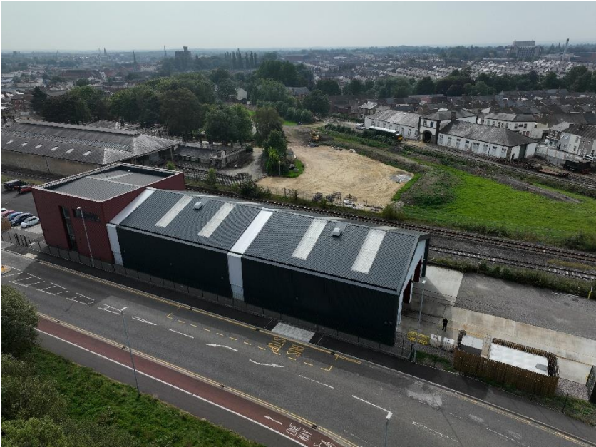
Aerial view of the new works
