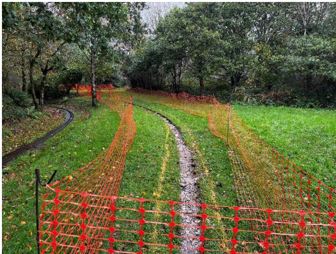
Initial removal of the old track pictured on 29 th October 2023
